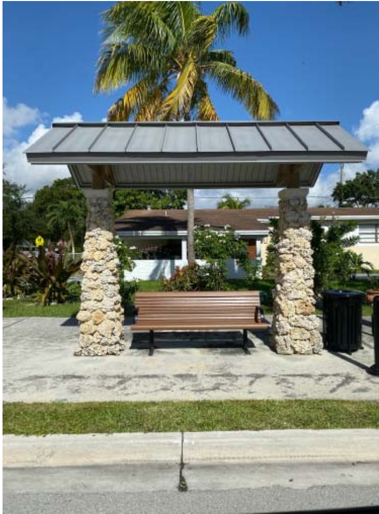
Pressure cleaning of one (1) standalone Bus Shelter
