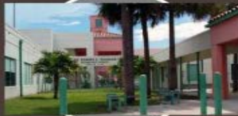
DR. EDWARD L. WHIGHAM ELEMENTARY SCHOOL 21545 SW 87 AVENUE
