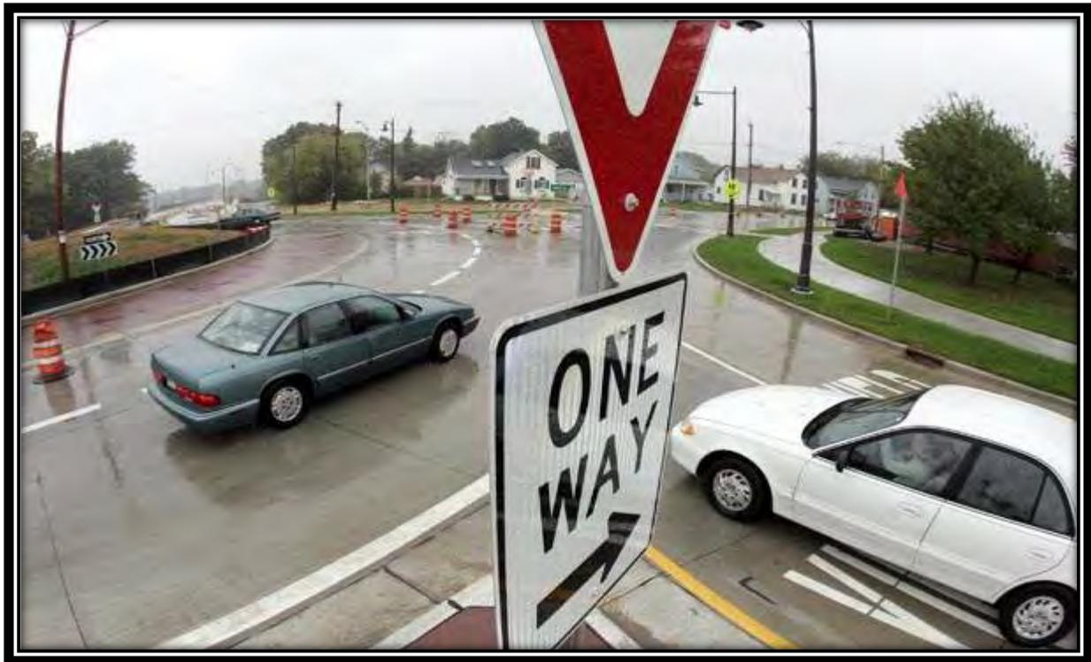
The modern roundabout is a type of raised intersection with no traffic lights. It is designed to reduce crashes and improve traffic flow. By understanding what a modern roundabout is and how it works, motorists, bicyclists and pedestrians can travel through intersections easier and more safely.
